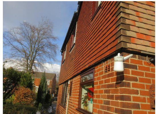
Photo taken from No 10 facing showing windows in side elevation
